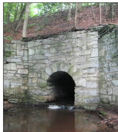
Arch-type railroad crossing (SC-02) may prevent fish passage and is suffering from downstream scour evidenced by the large pool shown in the photograph.
