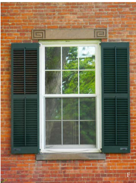
Fig. A, C: 12/12 double hung windows Fig. B: 6/6 double hung windows Fig. D: decorative palladian window Fig. E: bow window Fig. F: proper shutters on a 6 over 6 double hung window
