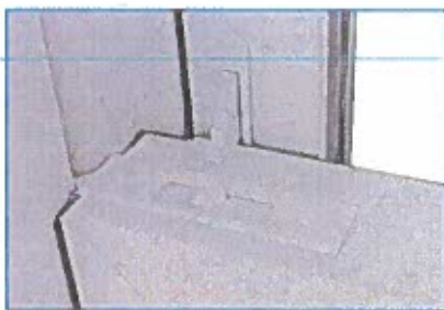
Vent Stop, when deployed, will limit sash travel to allow for ventilation.
