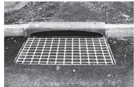
Figure 25. Bike Friendly Catch Basin Grate
