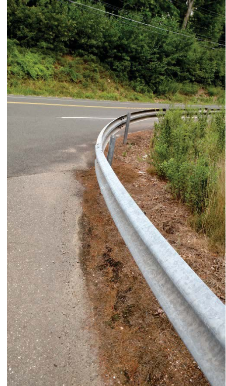
Figure 12. Loose Guard Rail
