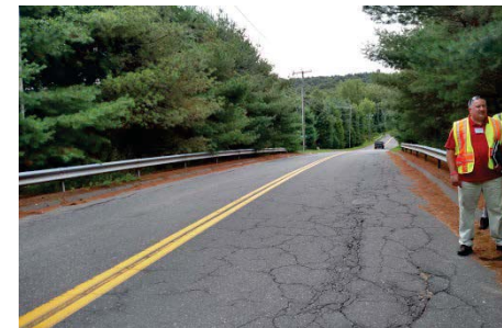
Figure 13. Poor Pavement Quality of Old Cathole Road
