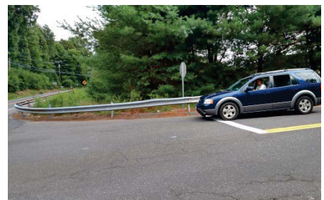
Figure 17. Stop Bar At Old Cathole Road Set Back Far
