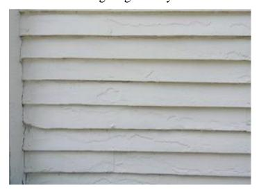
In most instances, total paint removal is not recommended or necessary. If paint is entirely removed a new coating should be reapplied to the exposed surfaces. Among the most destructive methods of paint removal is sandblasting which has become popular today as a 'quick and easy' way to remove paint. However, it is highly inappropriate for the Historic District, and alternative methods should be used.
