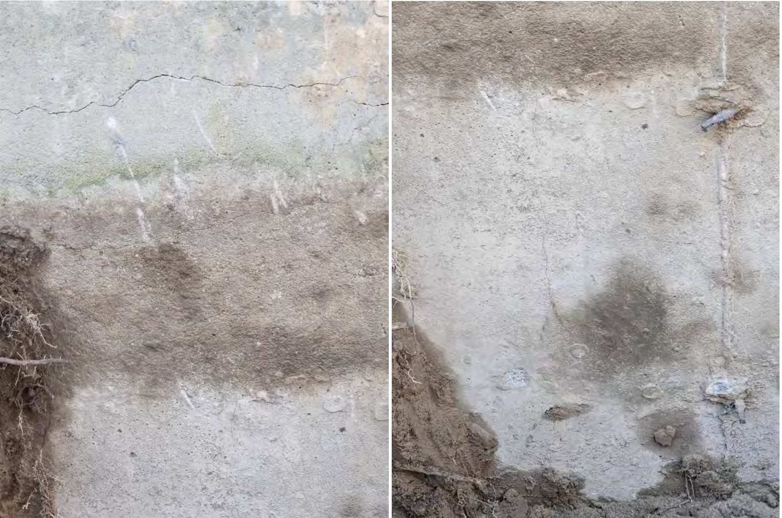
Eastern Foundation Wall (Vertical Crack with Horizontal Crack at the Top)
