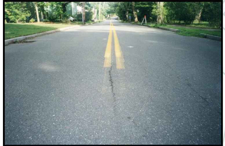
Routine Maintenance Condition (PCI 83-90)
