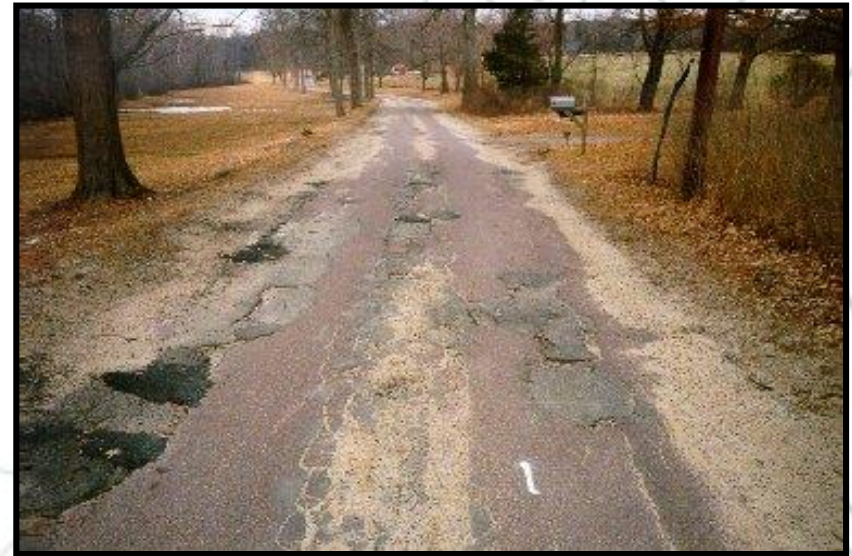
Base Rehabilitation Condition (PCI 0-55)
