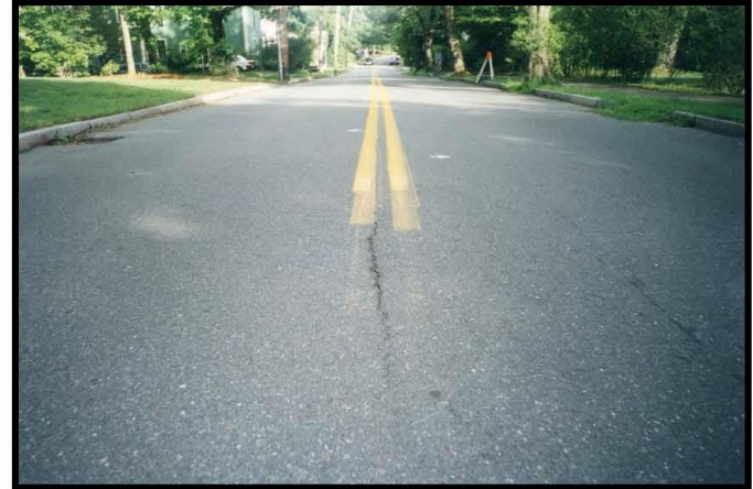
Routine Maintenance Condition (PCI 83-90)
