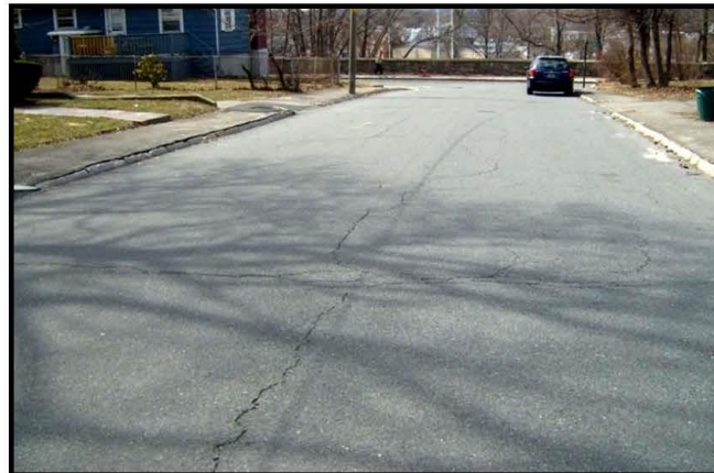
Preventive Maintenance Condition (PCI 71-82)
