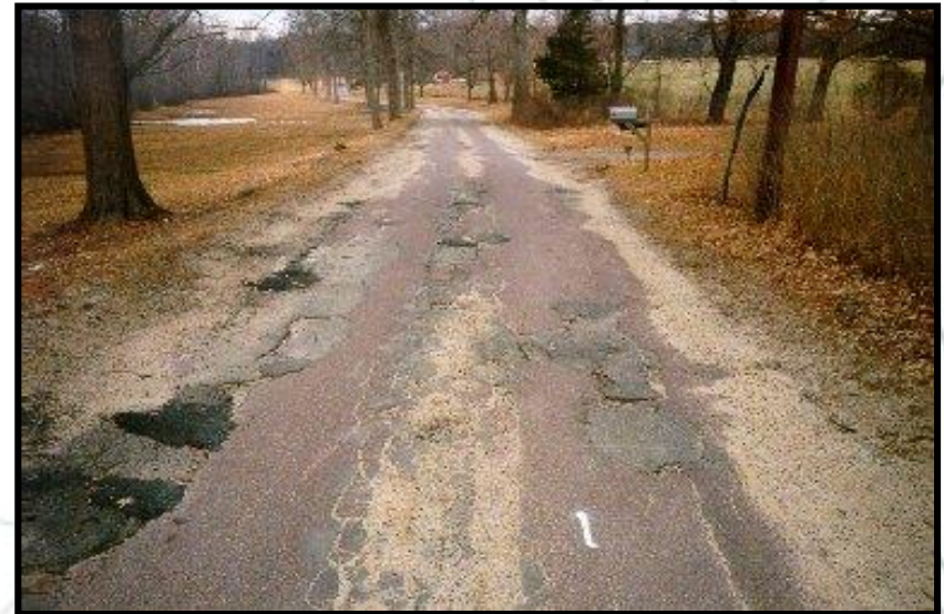
Base Rehabilitation Condition (PCI 0-55)
