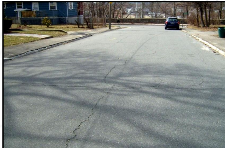
Preventive Maintenance Condition (PCI 71-82)
