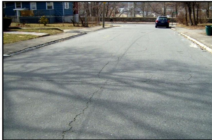
Preventive Maintenance Condition (PCI 71-82)
