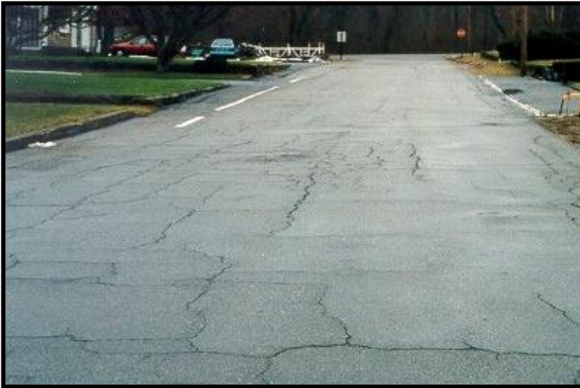
Structural Improvement Condition (PCI 56-70)
