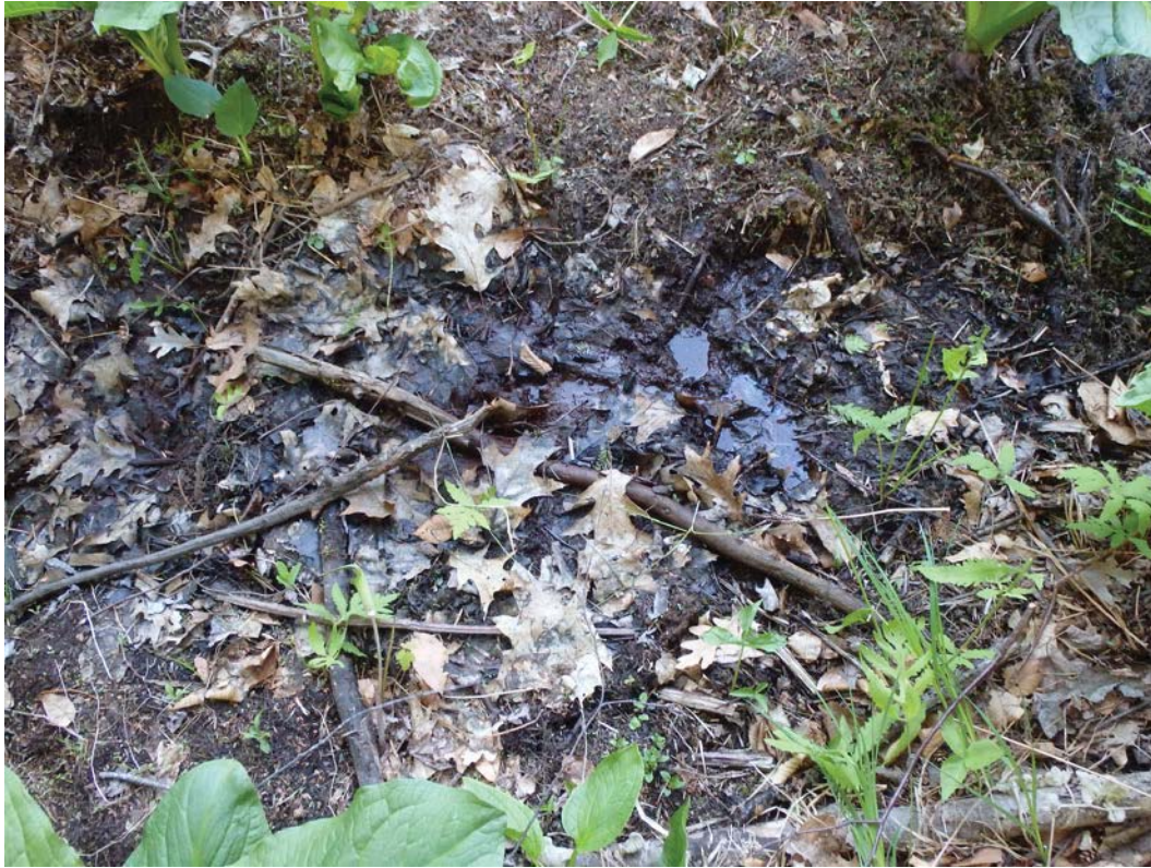
23. Minimal seepage at the embankment toe
