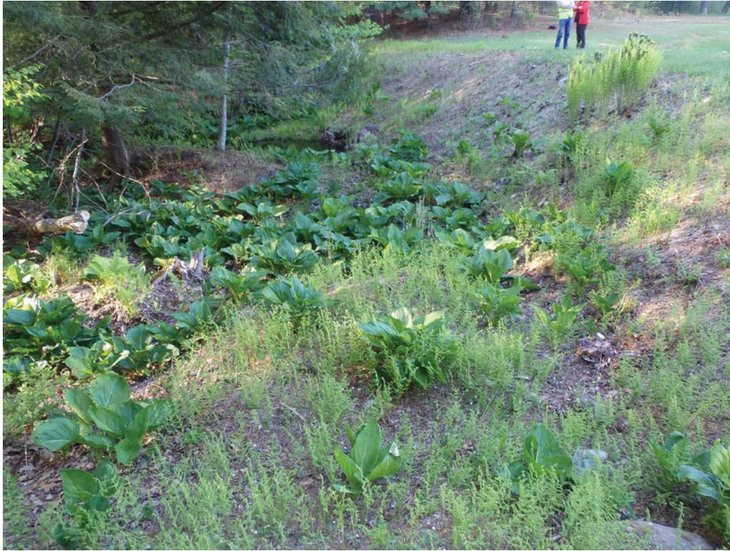
21. Skunk cabbage on lower downstream slope and foundation area indicative of seepage
