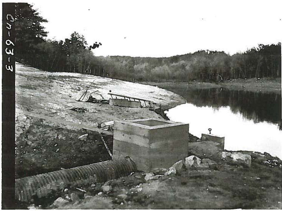
Above photo shows "gate" which allows one to lower pond-
