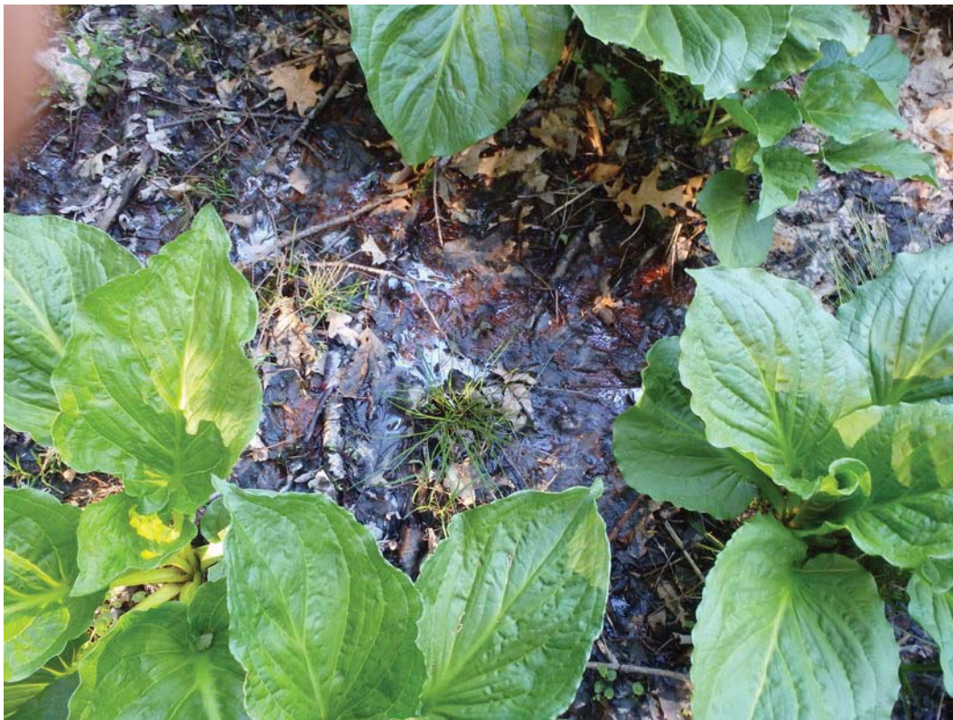
22. Close up of foundation soil surface downstream of embankment showing moisture at surface
