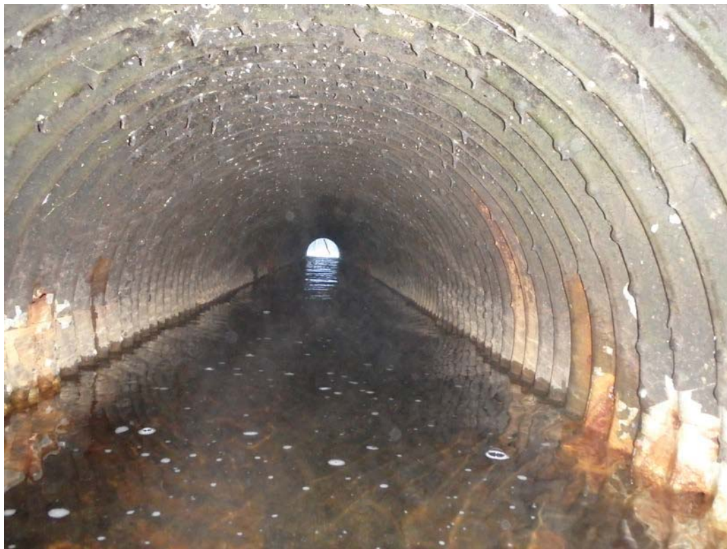
18. View of outlet conduit – note areas of corrosion
